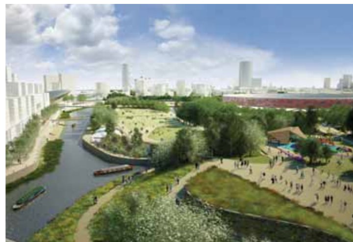
View south from the centre of the Legacy Park, showing the Stratford Waterfront neighbourhood to the left
